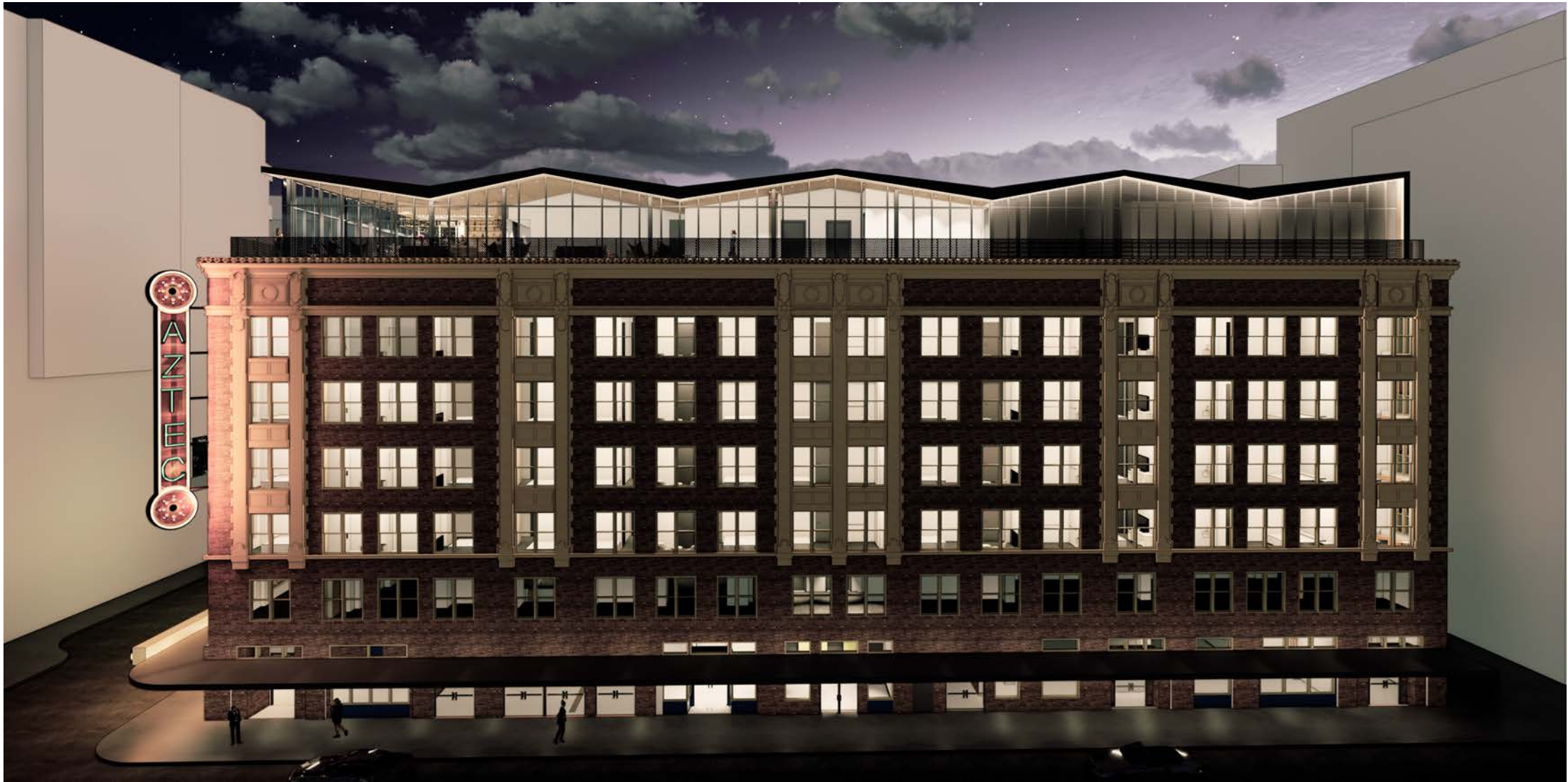
ELEVATION PERSPECTIVE ILLUSTRATES ALIGNMENTS TO EXISTING COMMERCE STREET FACADE ELEMENTS. ROOF PITCHES, RAILING, LOUVER SCREEN, AND GLAZING
